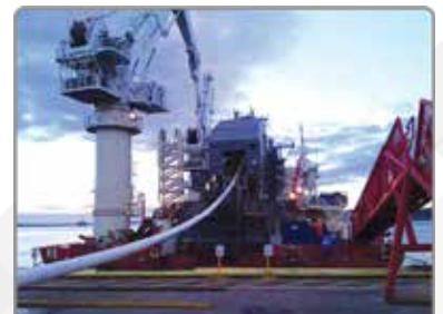
Completed electrically heat-traced pipe-in-pipe being reeled onto the pipelay vessel.
